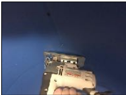
Figure 31 Cut the remainder of the hole with a jig saw
