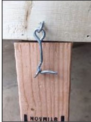
Figure 12 Make certain the hook and eye fit and create
