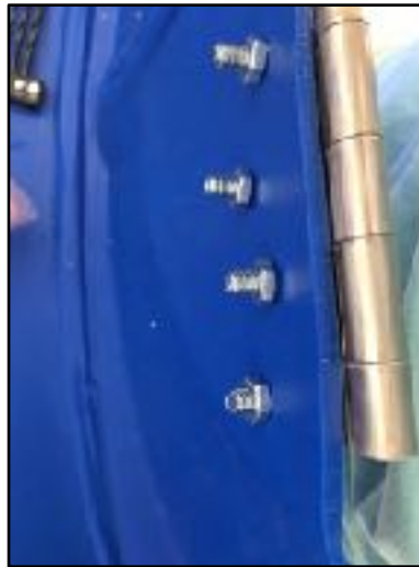
Figure 21 Secure 4"inch door hinge into place with nuts and bolts
