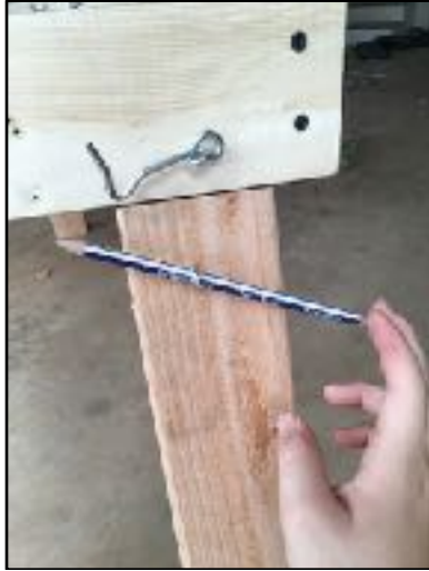
Figure 11 Screw the eye into the leg. a secure leg.
