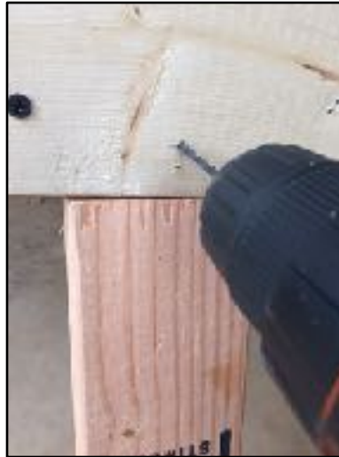
Figure 8 Create starting hole with a small drill bit.
