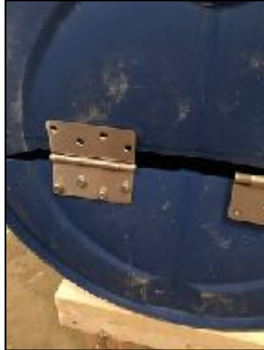
Figure 22 The barrel can be placed onto of the first to mark the drill holes properly.
