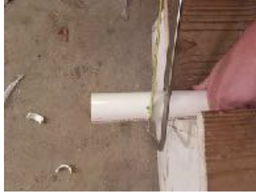
Figure 34 Cut the pip with a hacksaw.
