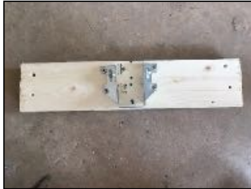
Figure 1 Screw the 2x4 hanger to piece B
